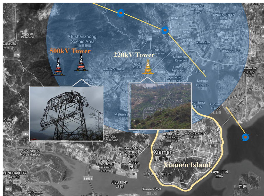
Fig. 2. Collapses of high-voltage transmission towers in Xiamen due to 2016 Typhoon Meranti.
